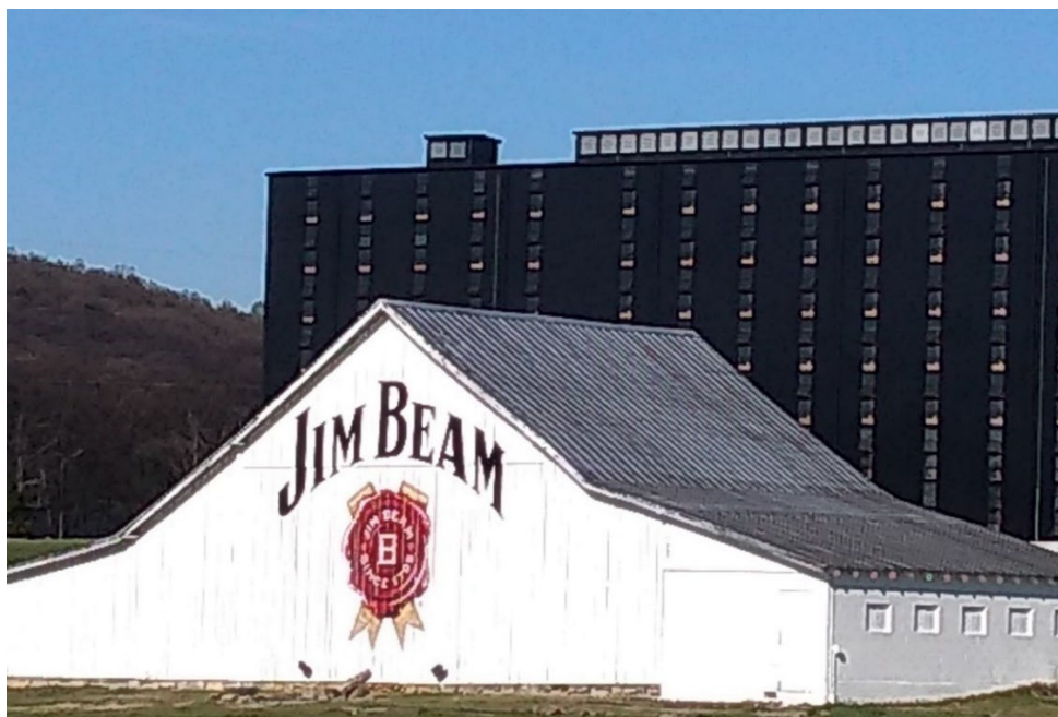
Figure 14. Jim Beam Suntory Warehouse. The black warehouse is like numerous new warehouses under construction. Court documents show that the LG & E Jim Beam Bullitt County Natural Gas Pipeline was originally planned solely to benefit Jim Beam's increased production, and when Jim Beam refused to pay the $20-$25 million project cost, LG & E and others developed a plan for rate payers to finance the project.
